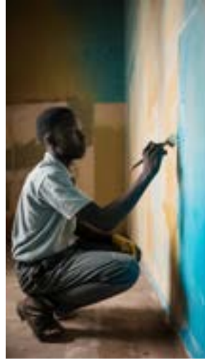
Applying oils or water-based polymers to protect surfaces from wear, moisture and UV light.
