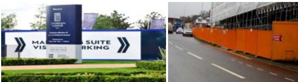
Fig. 5.13: Hoarding off the site prevents easy access.
