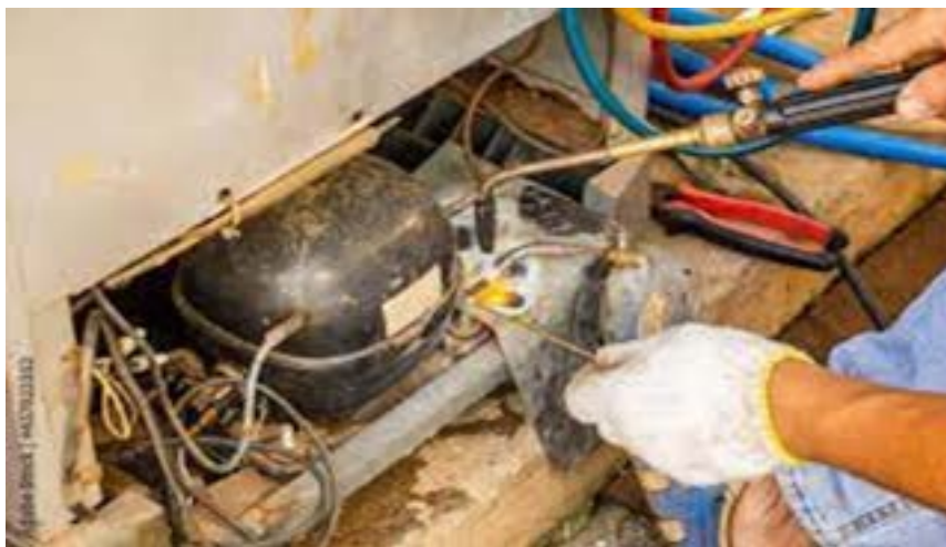
Fig. 5.15: Repair and maintenance with gas welding.
