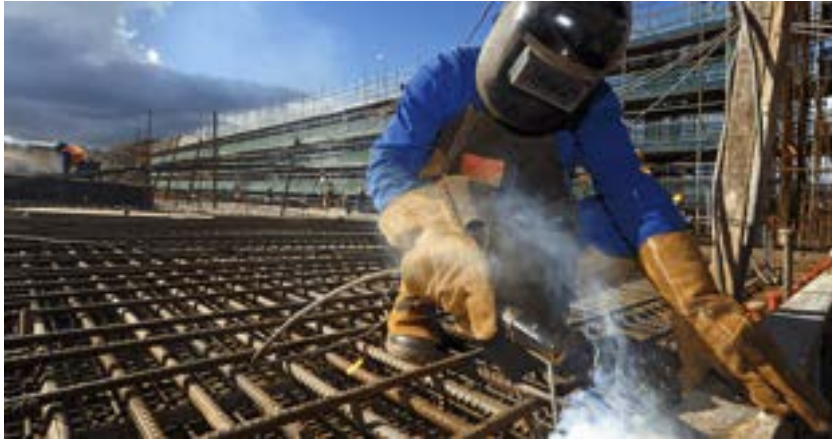
Fig. 5.24: Electric arc welding in the construction industry.
