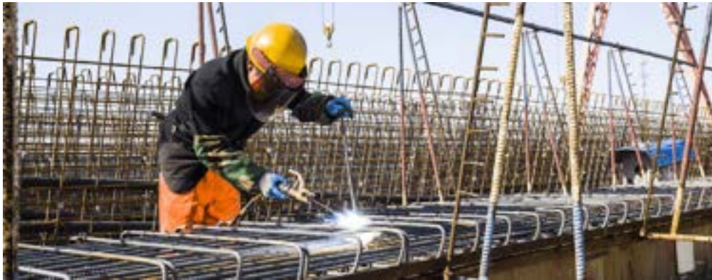
Fig. 5.16: Reinforcement fabrication with gas welding.
