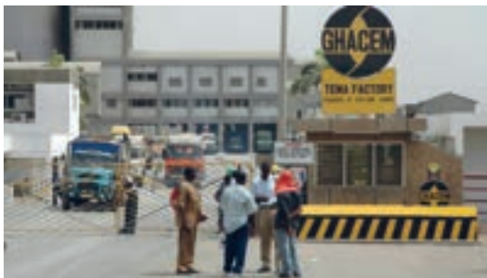
GHACEM Cement Production (Location of Industry)
