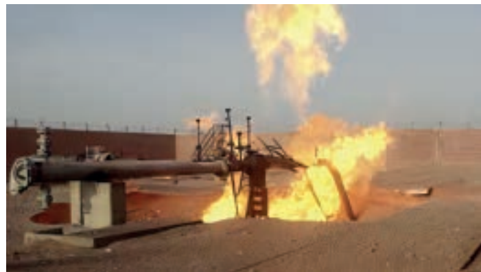
Figure 22: A picture of a pipeline explosions
