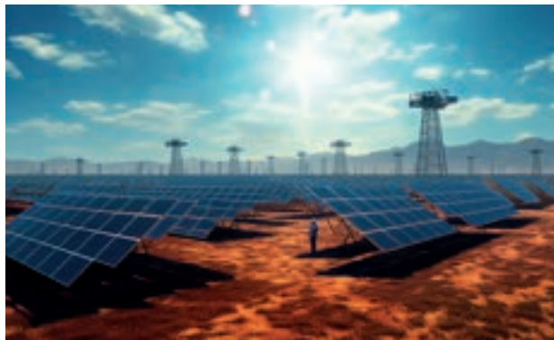
Figure 59: A picture of a Solar Generation Station
