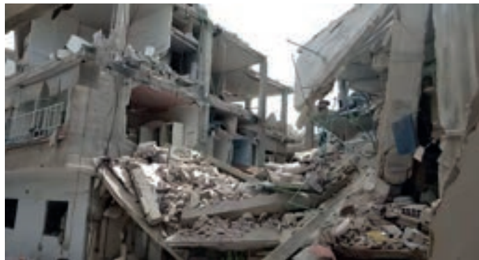
Figure 18: A picture of a structural failure
