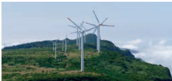
Figure 60: A picture of a Wind Energy Turbine
