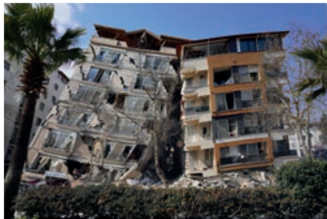
Figure 27: A picture of a collapsed building
