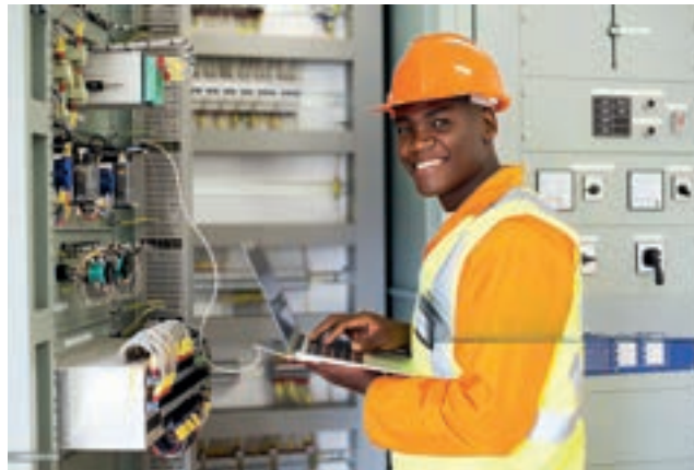
Figure 15: A picture of an electrical and computer engineer
