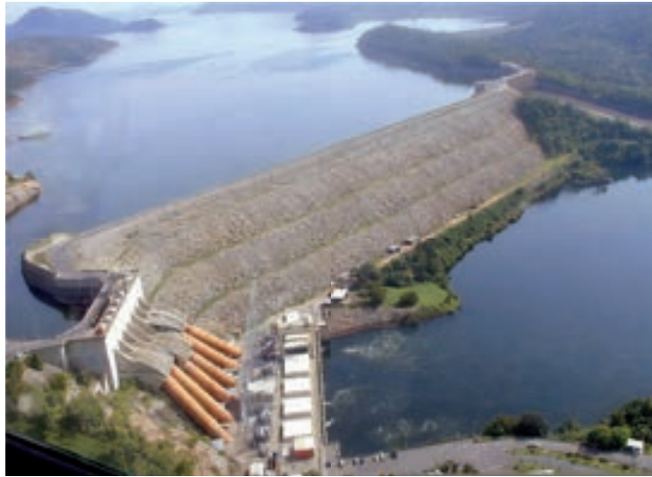
Figure 61: A picture of a Hydro Energy Generation Station
