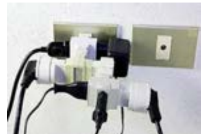
Figure 24.2: overloaded sockets
