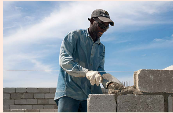
Fig. 1.3.4: Mason at work at a construction site.
