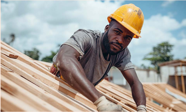
Fig. 1.3.5: A carpenter framing a roof.
