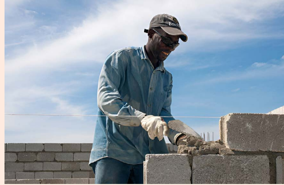
Fig. 1.3.4: Mason at work at a construction site.
