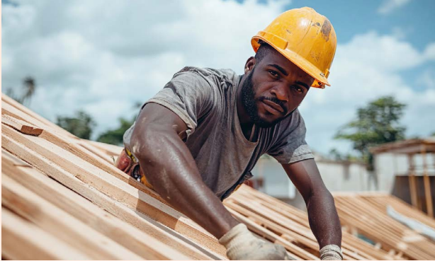
Fig. 1.3.5: A carpenter framing a roof.
