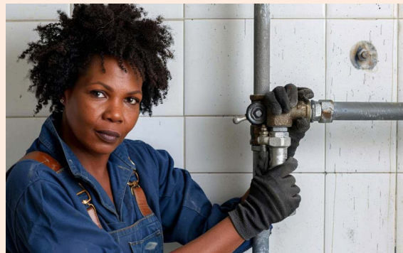
Fig. 1.3.7: Plumber at work
