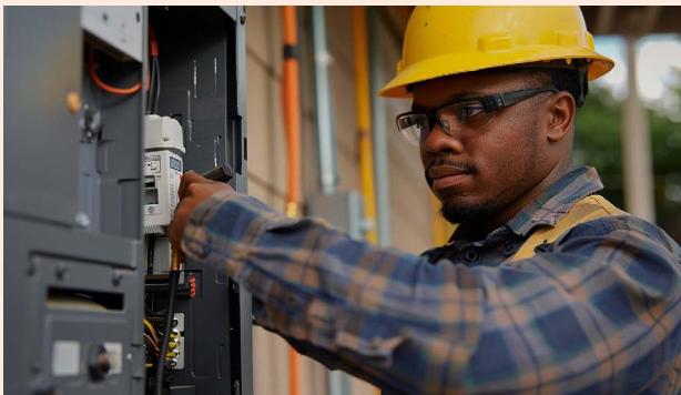
Fig. 1.3.6: Electrician at work.
