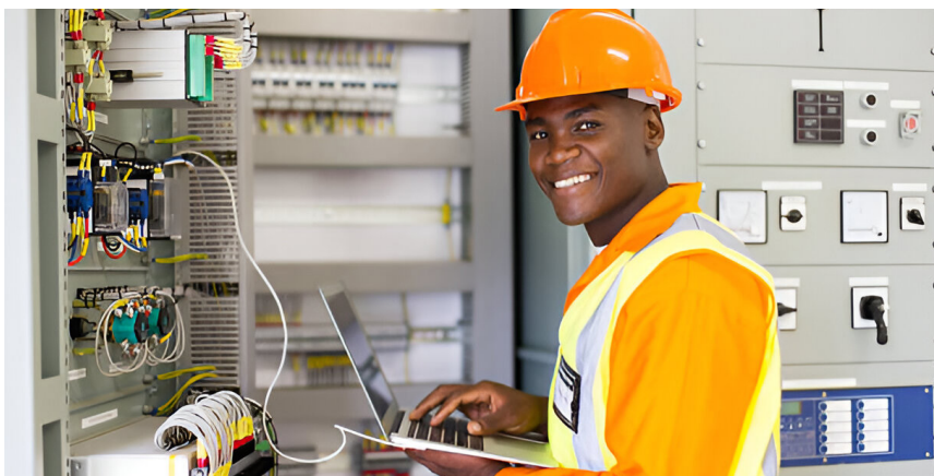
Fig. 1.3: A picture of an electrical engineer working inside a control panel.
