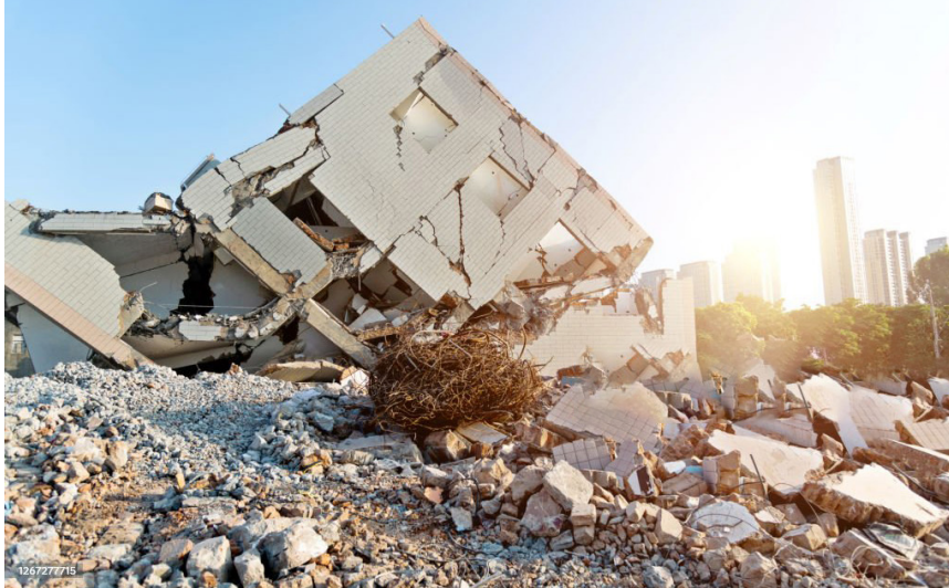
Fig. 2.10: A picture of a collapsed building
