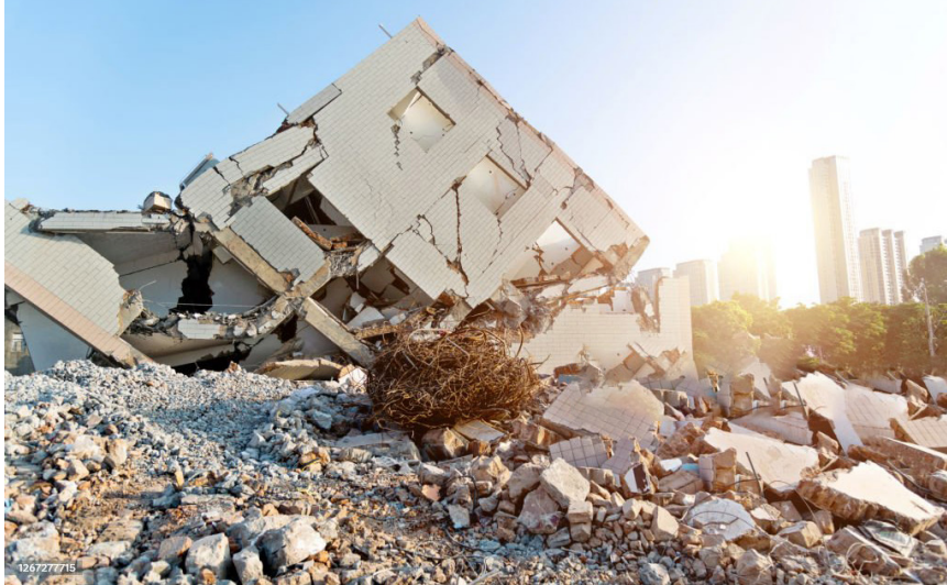
Fig. 2.10: A picture of a collapsed building
