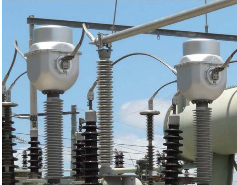
Fig 2.4.18: Distribution Feeder in a Substation
