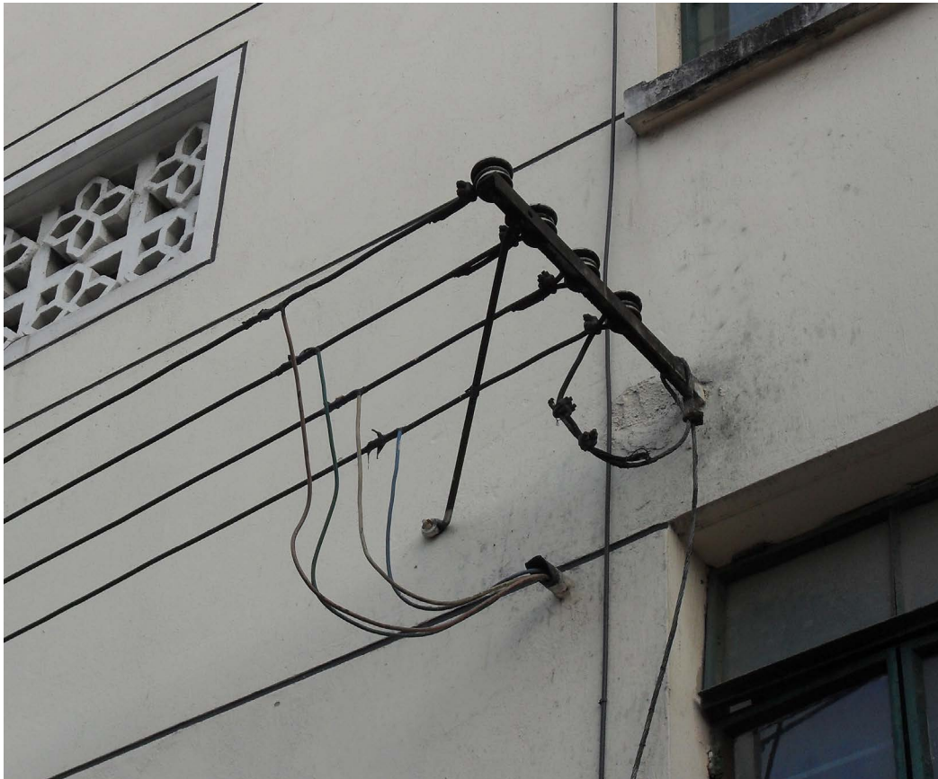
Fig 2.4.22: Three-phase distribution line
