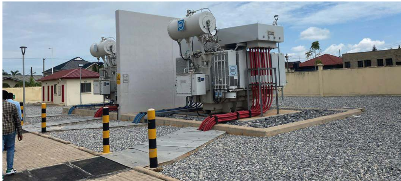
Fig 2.4.15: Power Transformer
