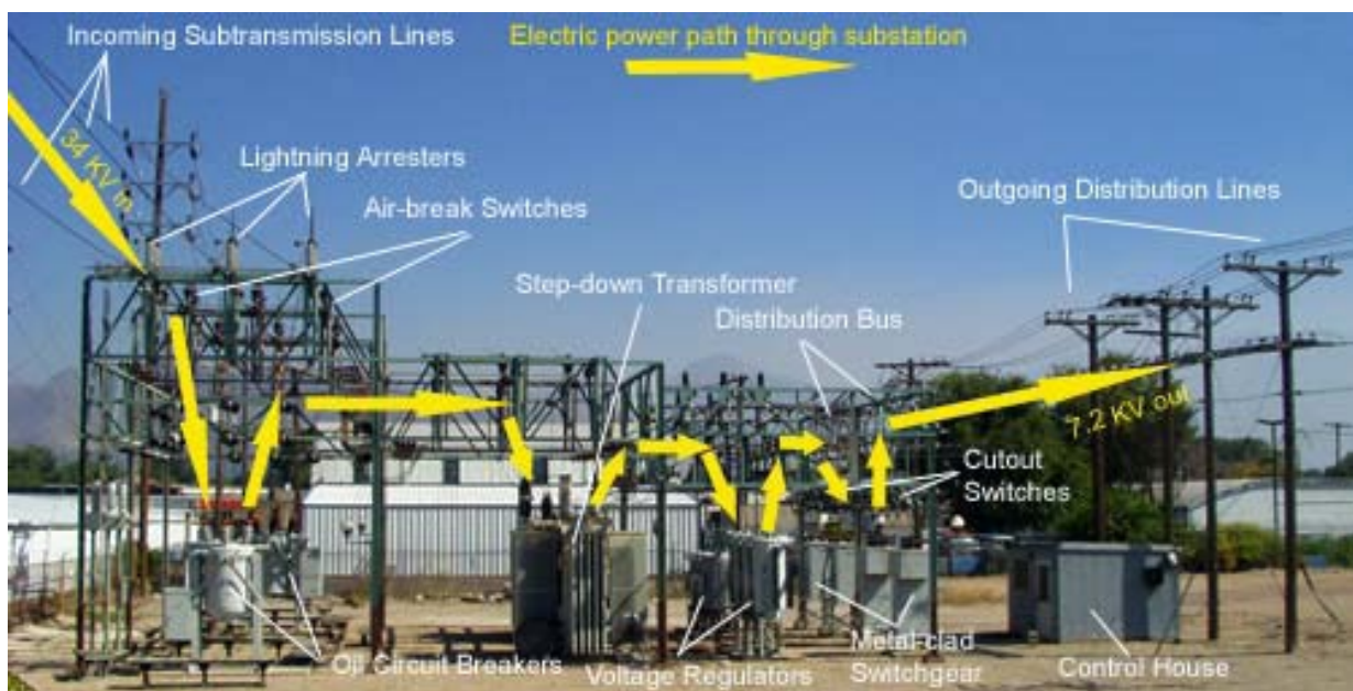
Fig 2.4.23: Electric power flow through Distribution Substation
