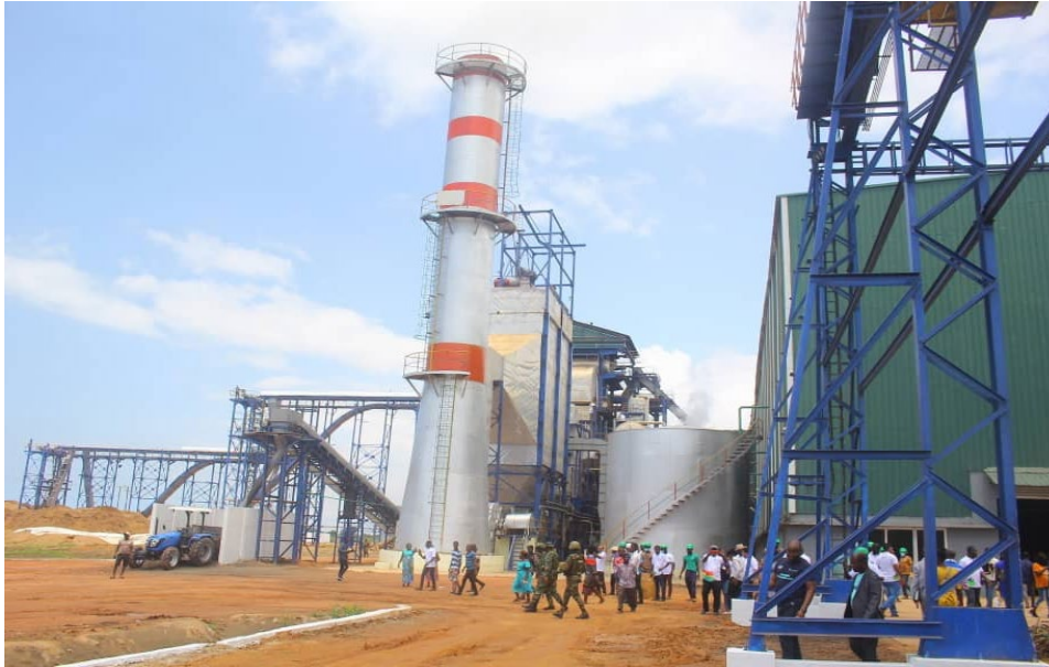
Fig. 4.2: Pictures Showing Some Capital Goods: Factory Buildings
