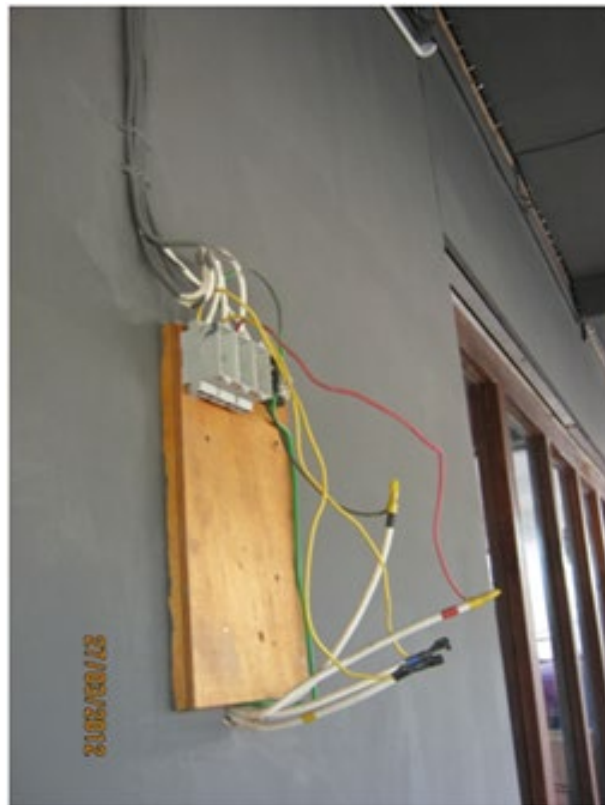
Fig.re 3.4.3: Picture of illegal wiretapping of electricity
