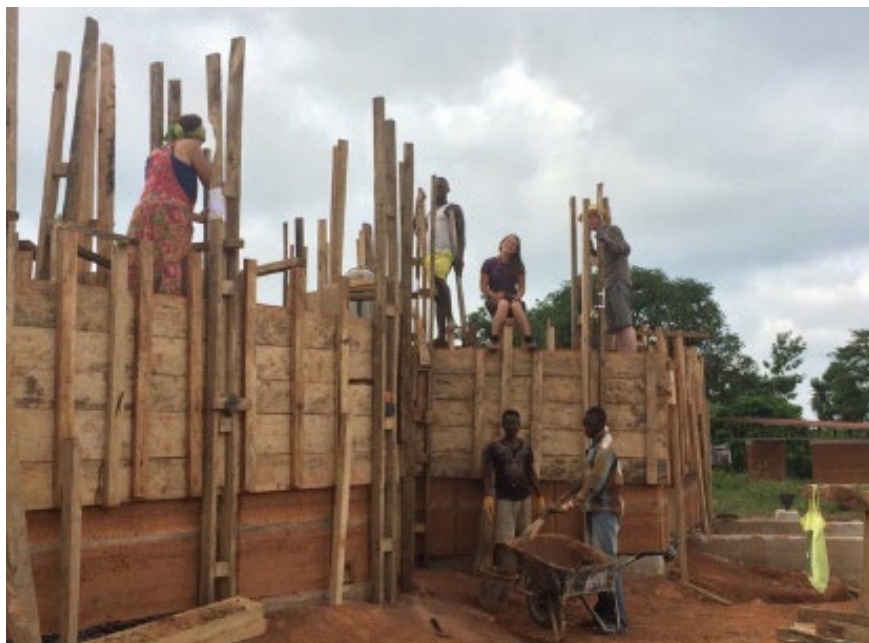
Figure 2.7: Construction of a Building
