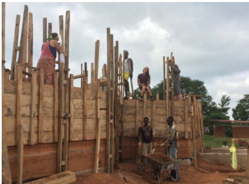
Figure 2.7: Construction of a Building
