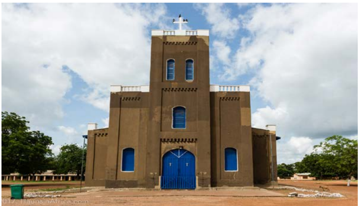
Fig. 10.7: Our Lady of Seven Sorrows Minor Basilica at Navrongo, a mud structure that has survived for more than 120 years.
