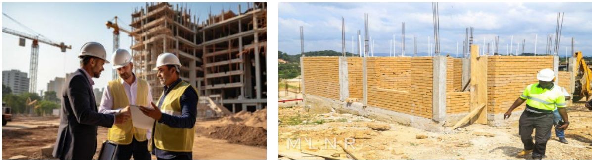
Figure 4.3.1: Professionals at Building construction sites
