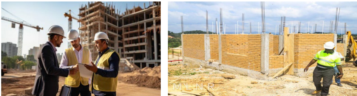
Figure 4.3.1: Professionals at Building construction sites
