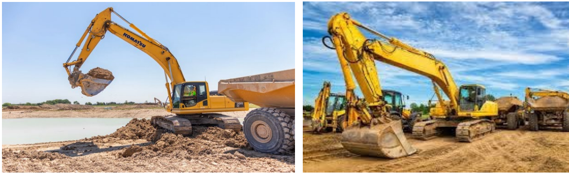
Figure 6.1.1: Excavators at the construction sites
