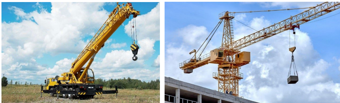
Figure 6.1.2: Cranes in use at the construction sites
