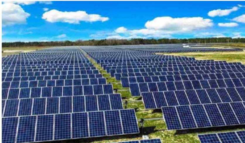
Fig. 5.12: A picture of solar panel
