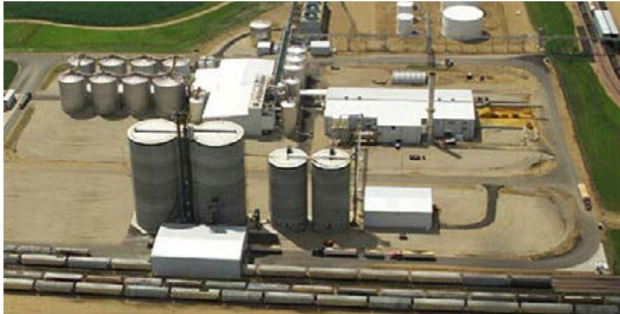
Fig. 5.4: A picture of a Biomass Energy Generation Station
