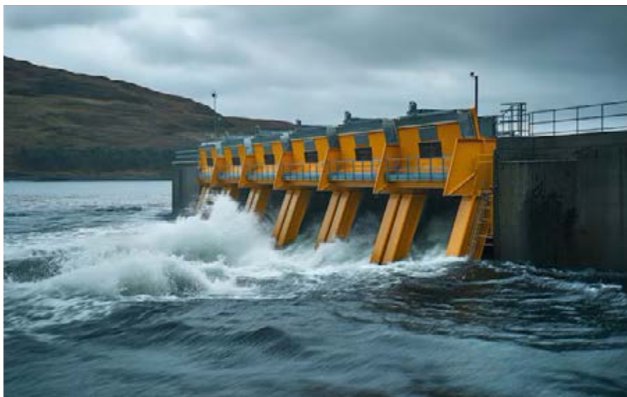
Fig. 5.6: A picture of a Tidal Energy Generation Station
