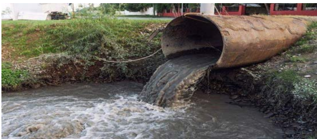
Fig. 12.9: Impure sewage water pouring into running water
