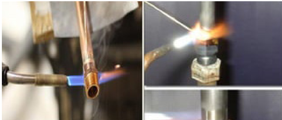
Figure 6.20: Hard soldering of pipes
