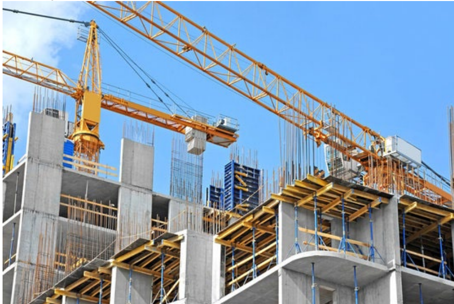
Figure 4: An image of a construction site
