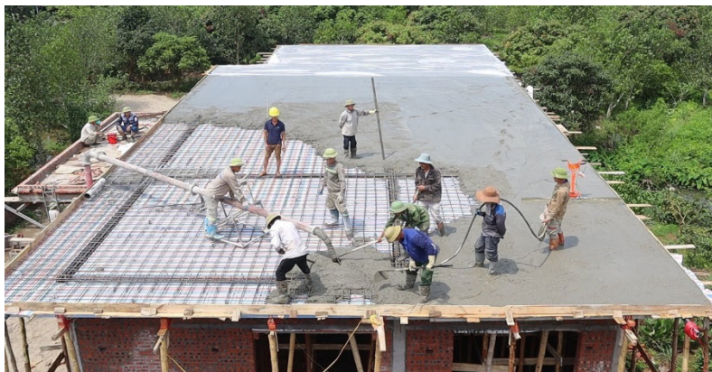
Figure 6.23: Concrete flat roof
