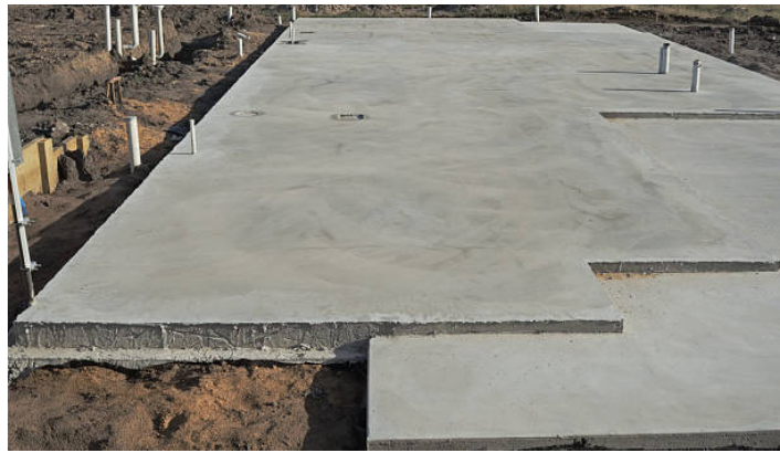
Figure 1.48: Oversite concrete floor slab for substructure
