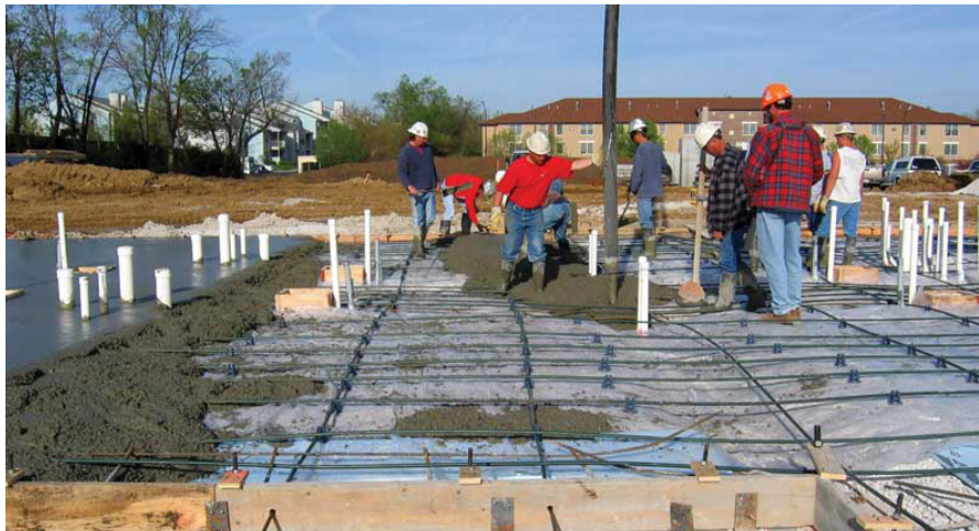
Figure 4.4: Solid Ground Floor slab with mesh reinforcement
