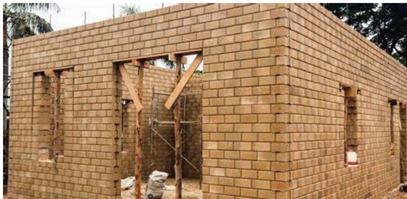
Figure 5.30: Load or Mullion wall
