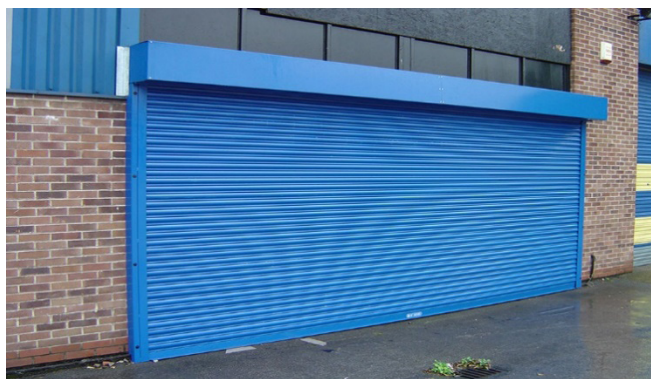
Figure 5.37: Rolling shutter door
