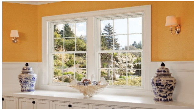
Figure 5.42: Double hung window
