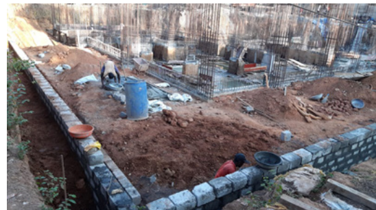
Figure 3.3: Block footings
