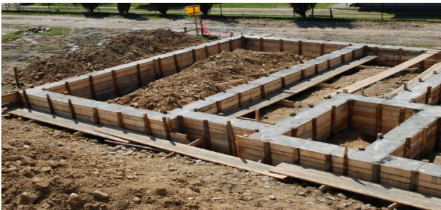
Figure 3.2: Concrete footings
