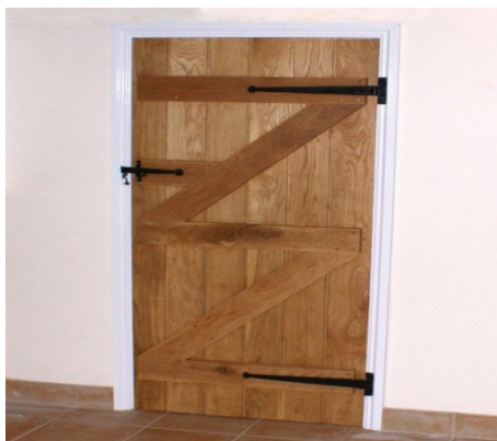
Figure 5.39: Ledged and braced door
