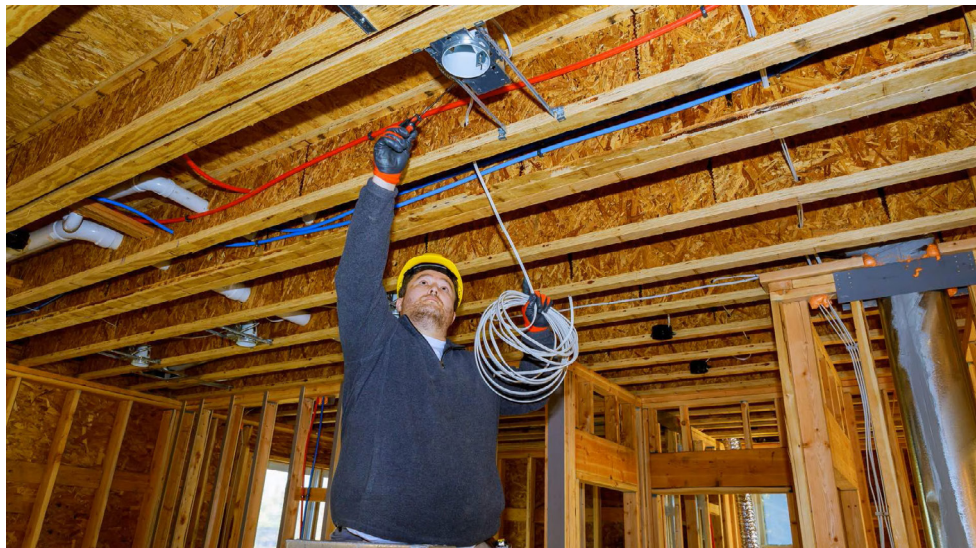
Figure 1.1: Wiring being carried out
