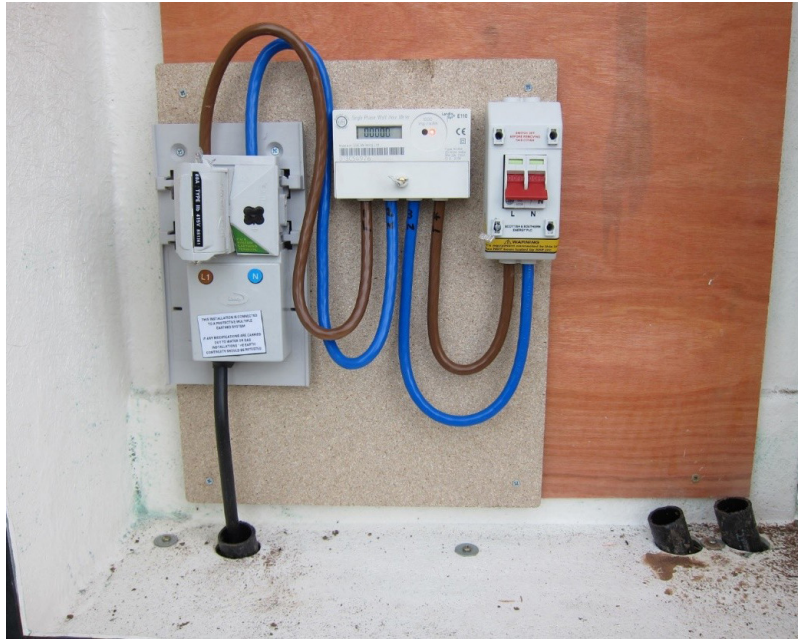
Figure 1.2: Wiring of supply- control equipment
