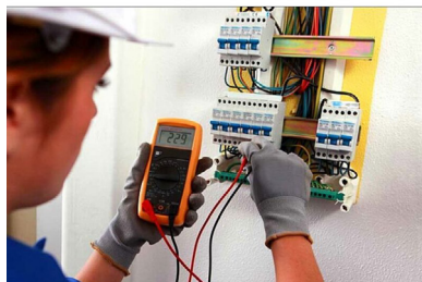
Figure 2.16: Testing of a circuit
