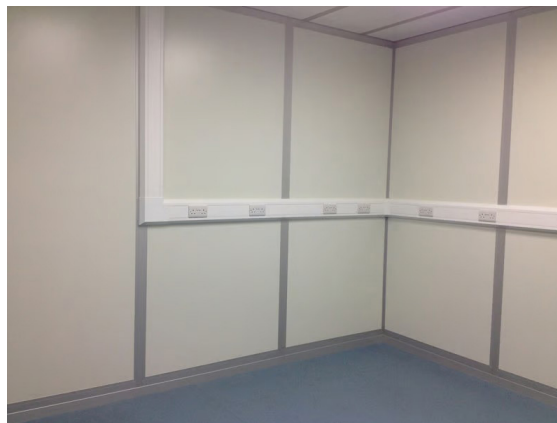
Figure 2.6: Trunking system
