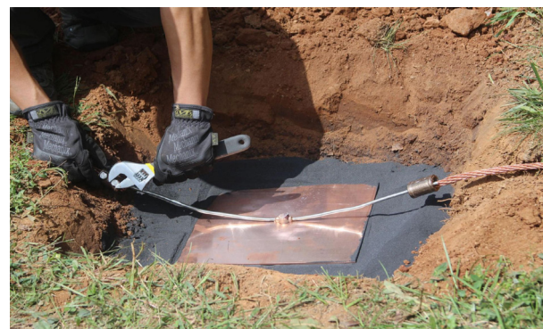
Figure 3.7: Plate earthing
