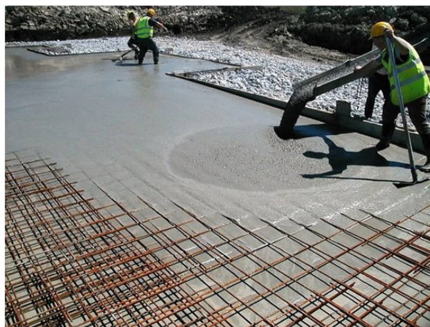
Figure 1.2.8: Compacting of the concrete slab
