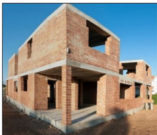
a Load-bearing wall
