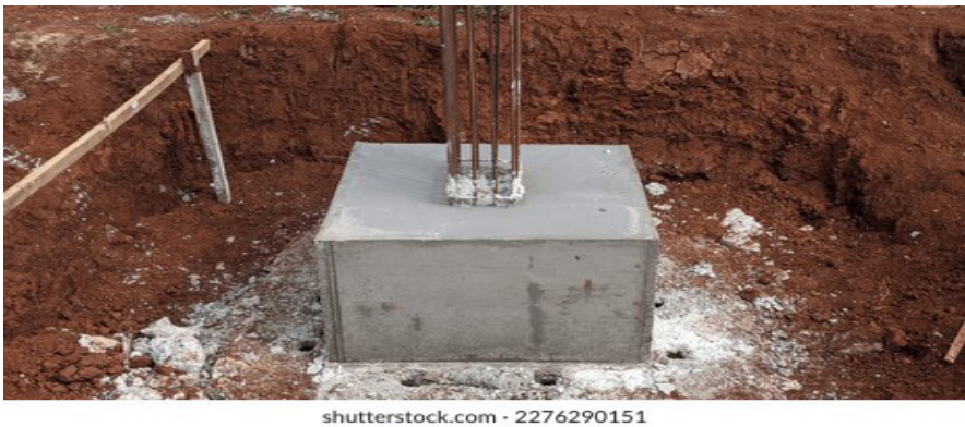
Fig. 3.10.2: An example of a foundation footing showing some of the elements
