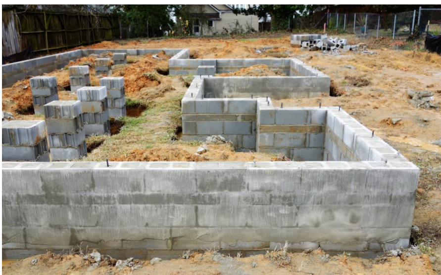
Figure 1.2.4: Example of block footings
