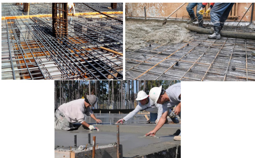
Figure 1.2.7: Levelling of concrete slab
