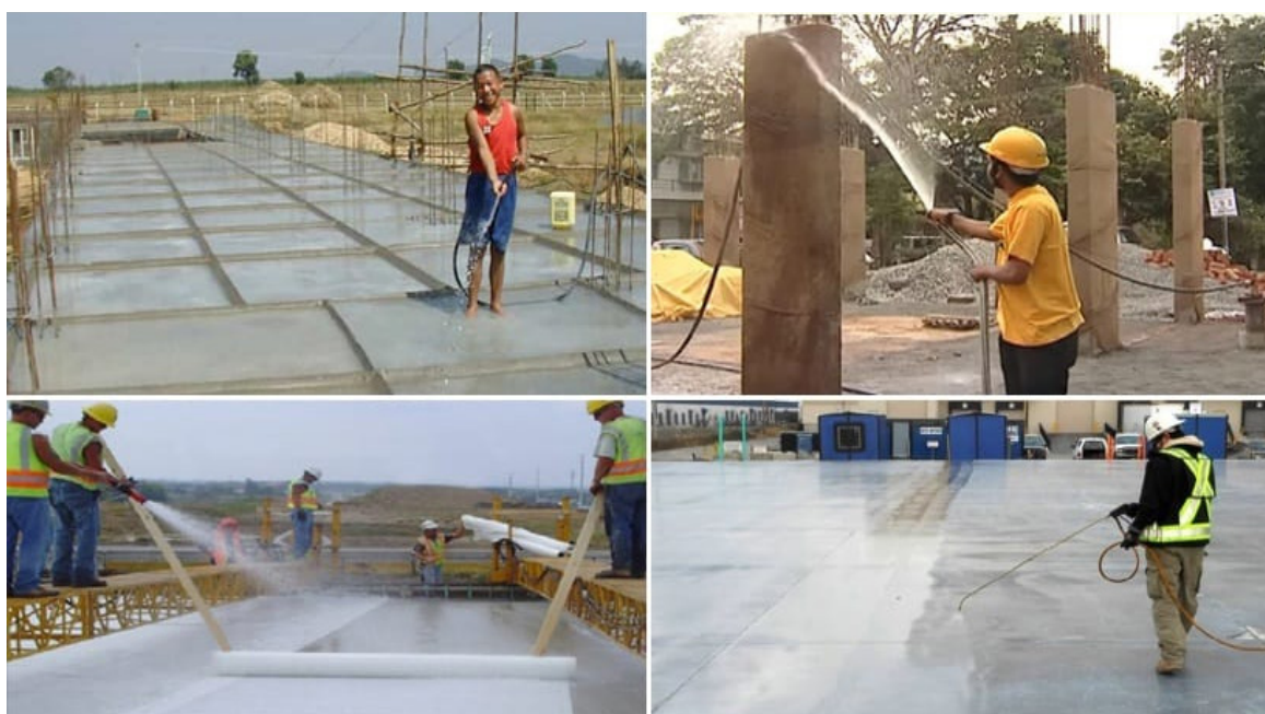
Figure 1.2.9: Curing of concrete slabs
