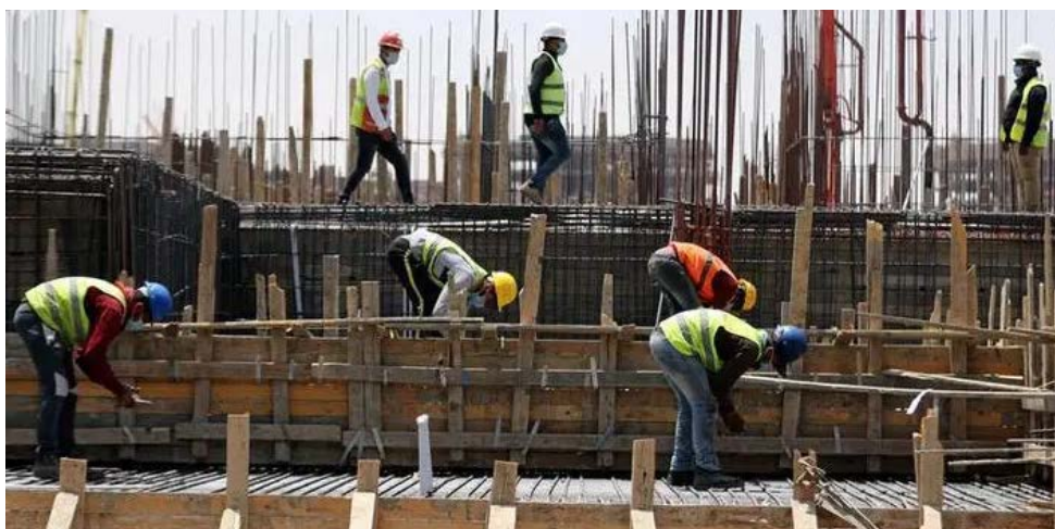
Figure 2.19: An image of a construction site
