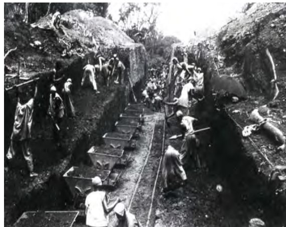
Force labour on a road construction site
