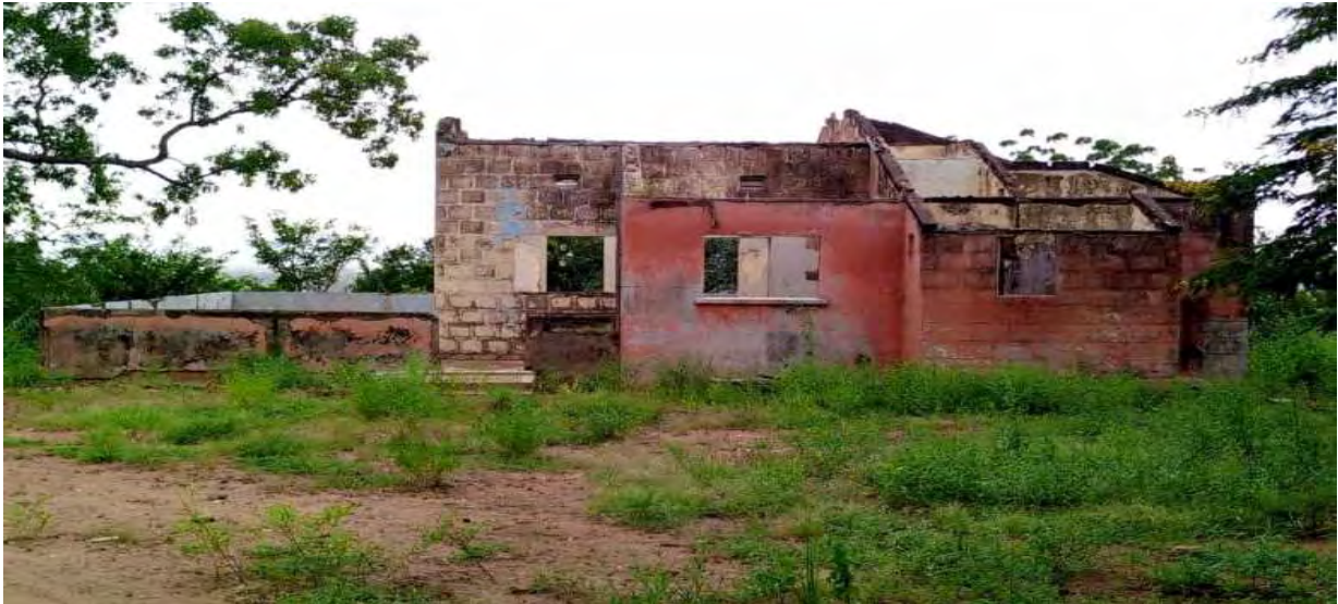
Figure 4.10: An old house at Karimenga in the North East Region of Ghana
