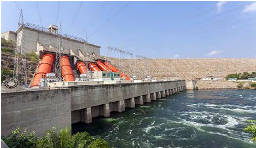
Figure 4.13: An image of the Akosombo Dam (opened in 1965)
