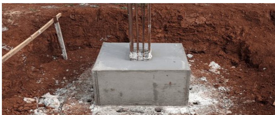
Fig. 3.10.2: An example of a foundation footing showing some of the elements
