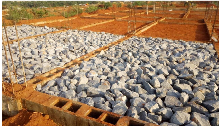
Figure 1.2.5: Example of hardcore filling at the construction site
