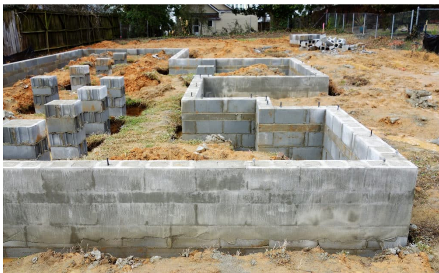
Figure 1.2.4: Example of block footings
