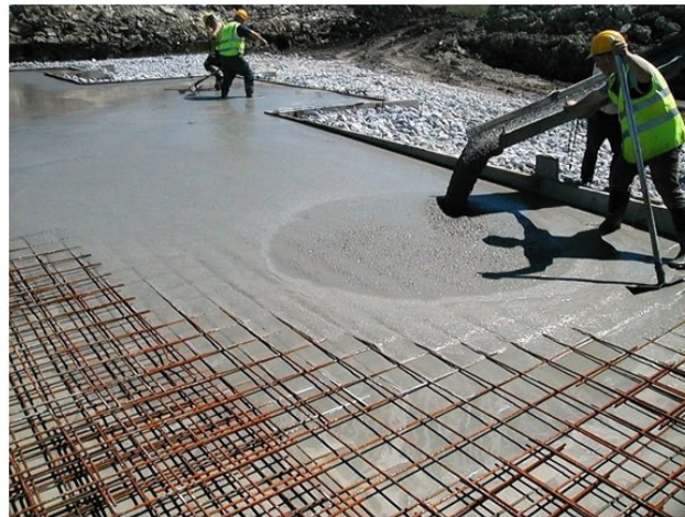
Figure 1.2.8: Compacting of the concrete slab
