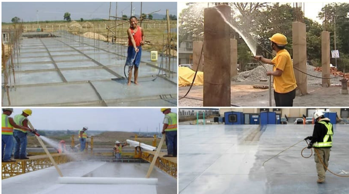
Figure 1.2.9: Curing of concrete slabs
