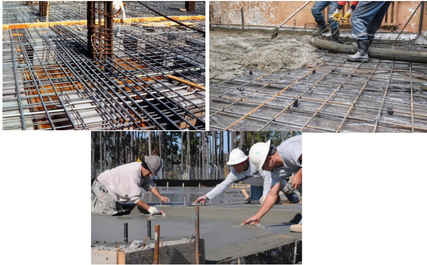
Figure 1.2.7: Levelling of concrete slab
