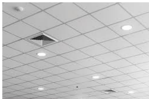
Figure 6.24.1: Suspended ceilings
