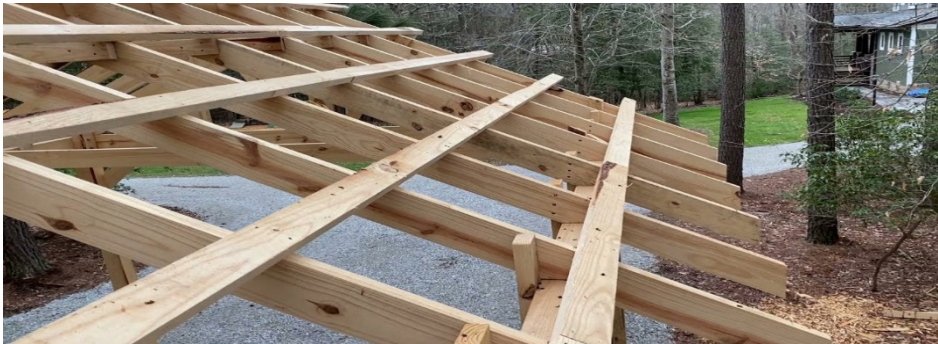
Figure 6.22.10: Typical positioning of rafters and purlins during roof construction
