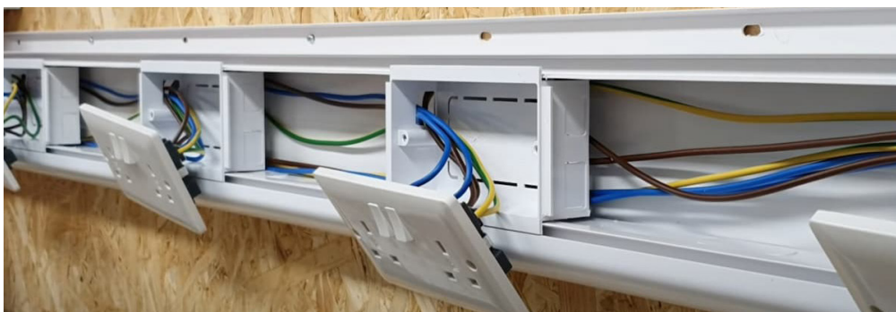
Figure 2.6.4: Example trunking showing sockets
