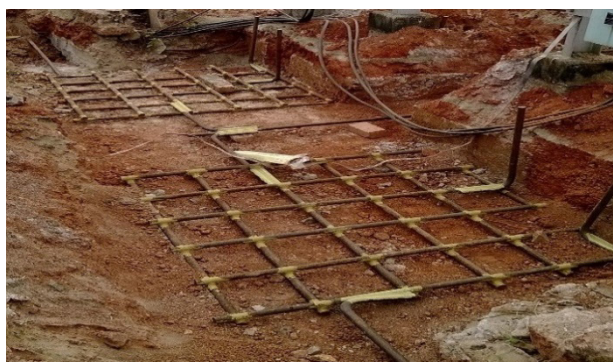
Figure 3.9.2: Pictures of earthing method using wire mesh
