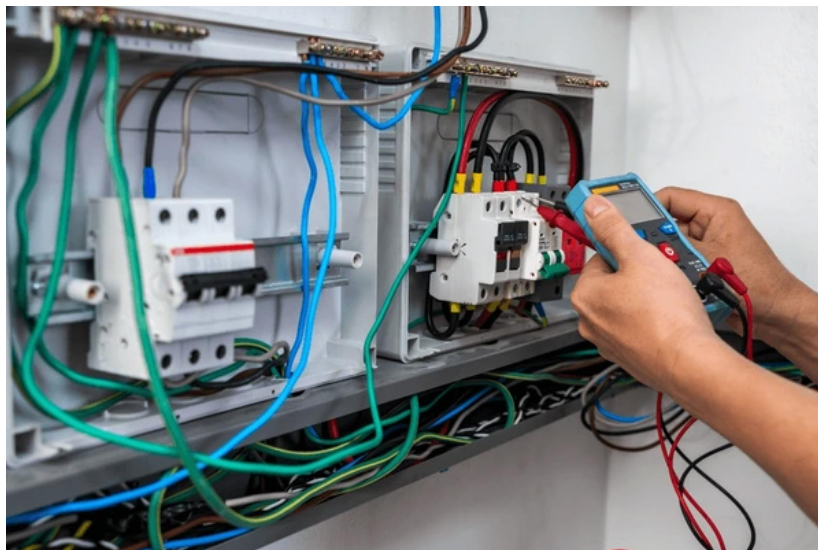
Figure 5.6: A picture of circuit breakers in combiner boxes
