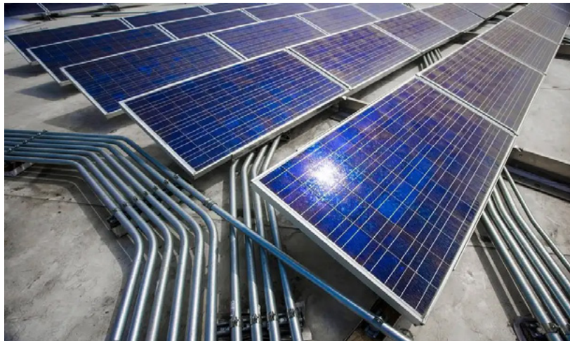
Figure 5.8: A picture of photovoltaic wiring
