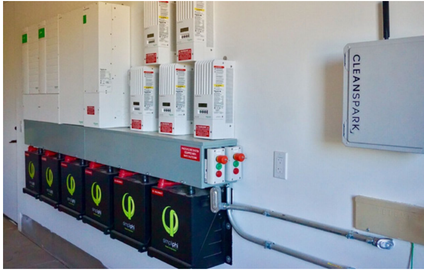
Figure 5.5: A picture of Photovoltaic batteries
