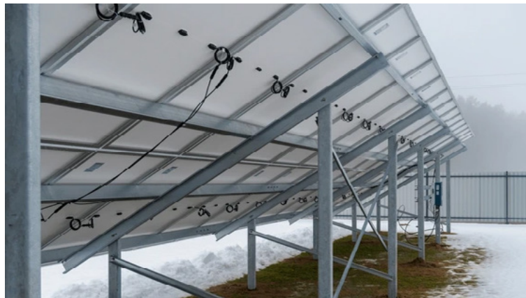
Figure 5.3: A picture of the PV module mounting system
