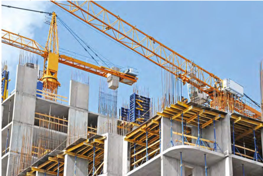
Figure 4: An image of a construction site
