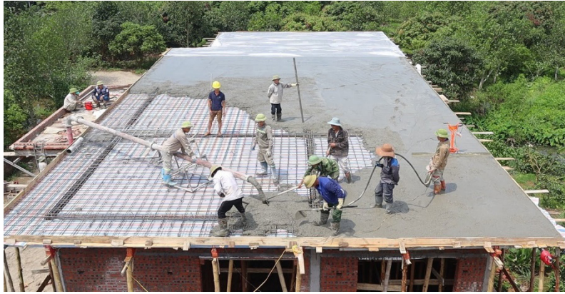
Figure 6.23: Concrete flat roof
