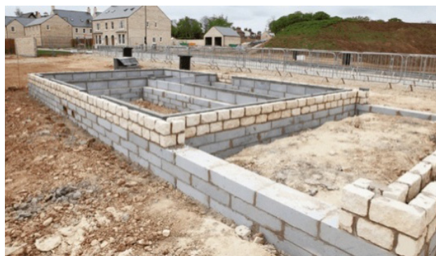
Figure 1.47: Foundation footing of a building
