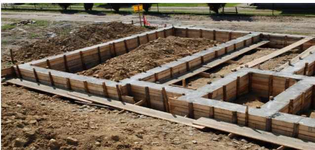
Figure 3.2: Concrete footings
