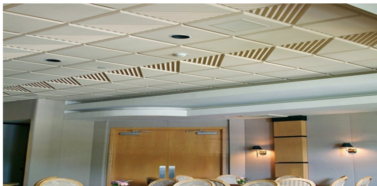
Figure 6.32: Acoustical ceilings
