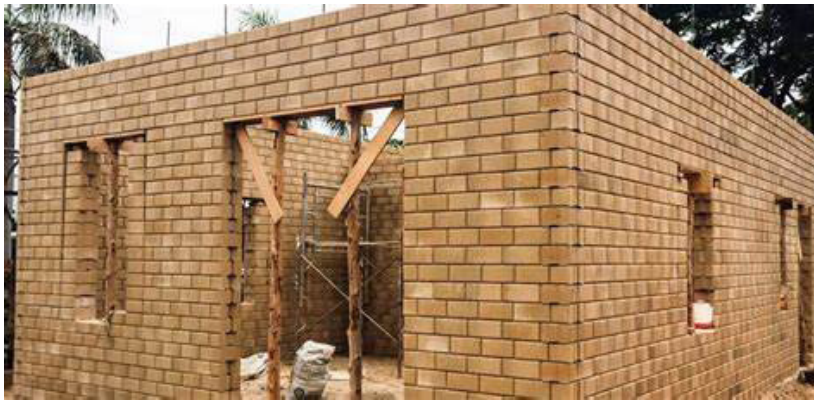
Figure 5.30: Load or Mullion wall
