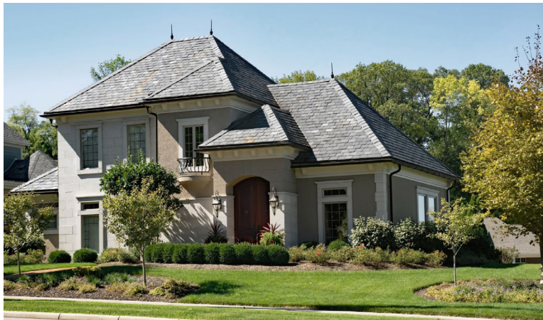
Figure 6.25: Hipped Roof
