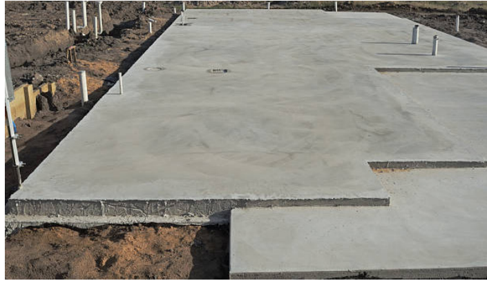
Figure 1.48: Oversite concrete floor slab for substructure
