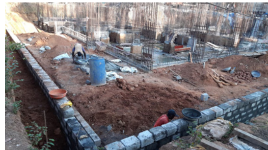
Figure 3.3: Block footings
