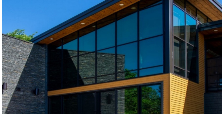
Figure 5.29: Curtain wall
