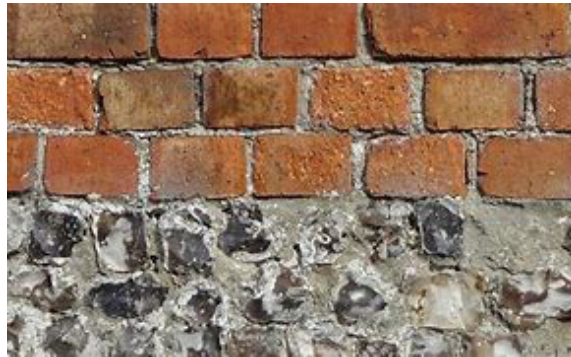
Figure 5.27: Solid wall
