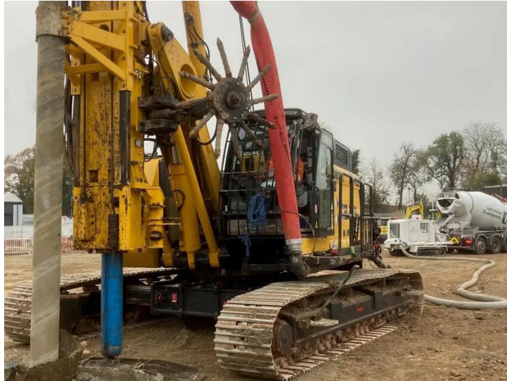
Figure 2.21: Drilling Pile
