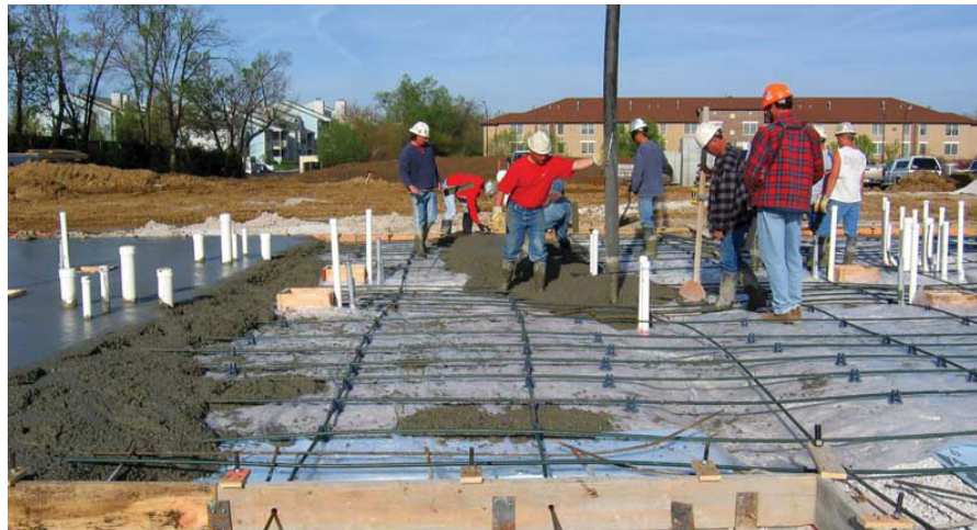
Figure 4.4: Solid Ground Floor slab with mesh reinforcement
