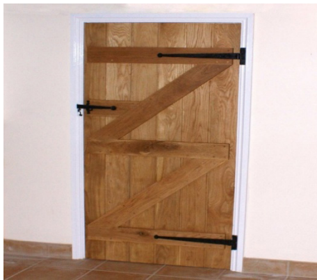
Figure 5.39: Ledged and braced door
