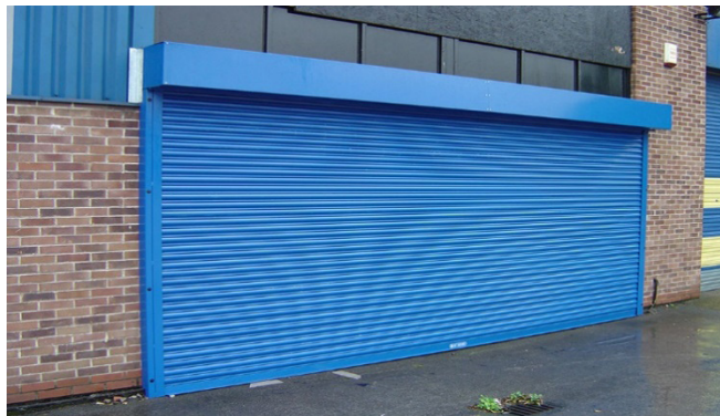
Figure 5.37: Rolling shutter door
