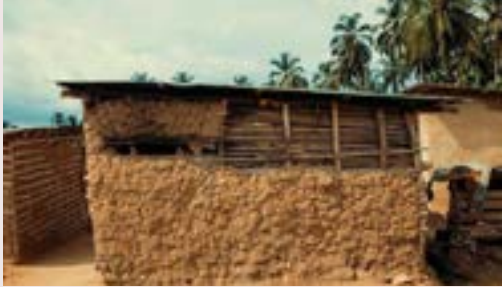
( Picture of a rural house in Ghana )
