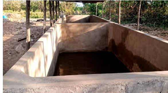
B. A completed rectangular concrete tank
