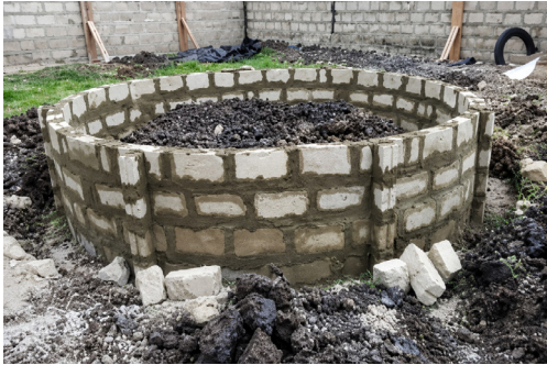
Figure 6.3: A. A circular concrete tank under construction
