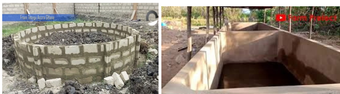
Figure 6.3 A: – A circular concrete tank under construction. B – A completed rectangular concrete tank
