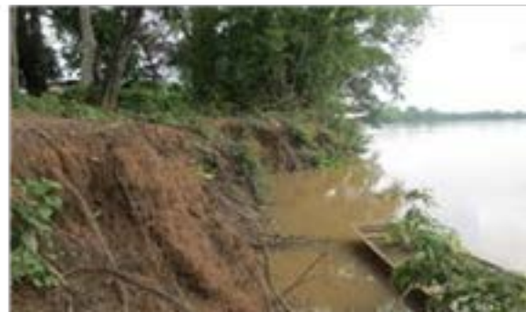
Figure 4.6 b: Riverbank erosion
