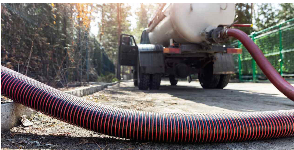
Figure 1.3.5: Example of waste disposal by a vacuum tanker or Sewerage tanker
