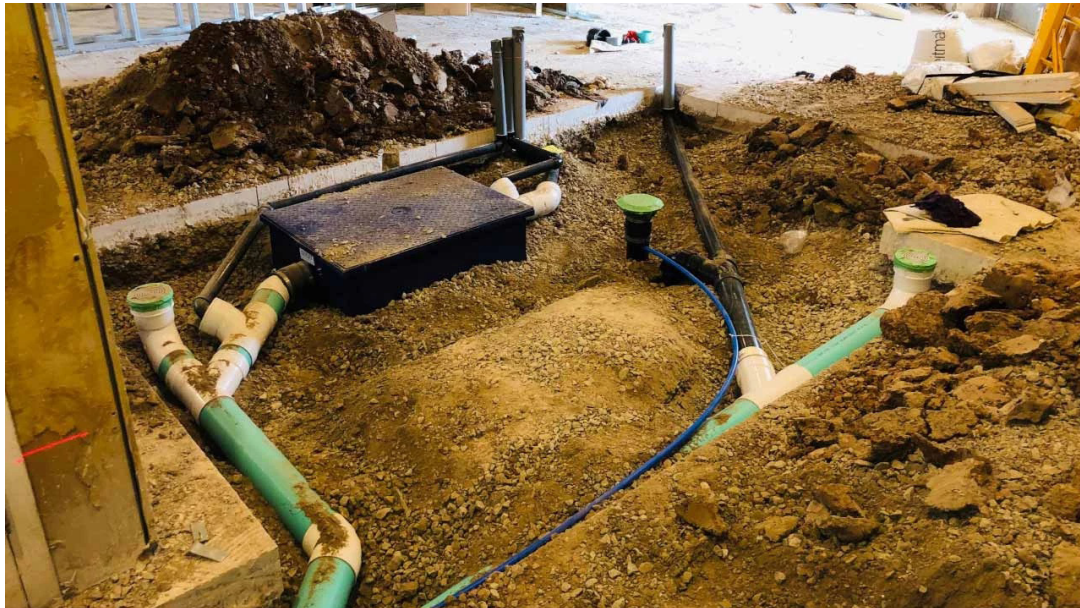
Figure 3.9.1: Example of laid waste pipes
