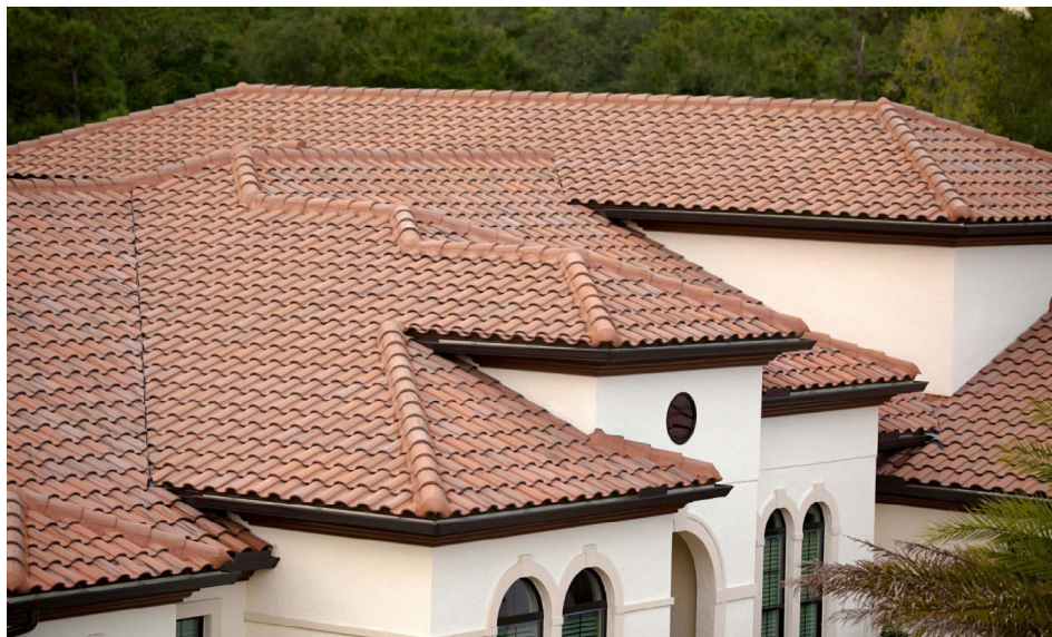
Figure 5.19.3: An example of a concrete tile roof
