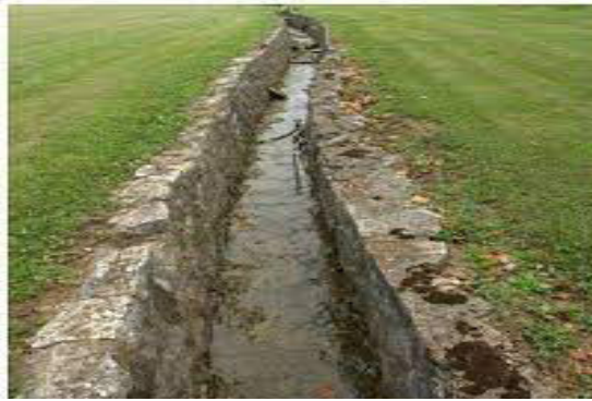
(A) Open surface drain system
