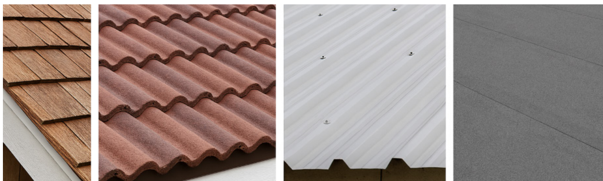
Figure 5.19.1: Example of shingle roof, concrete tiles roof, Corrugated aluminium roof and flat roof.
