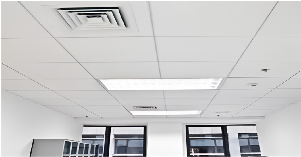
Figure 5.20.1: Gypsum board ceiling.
