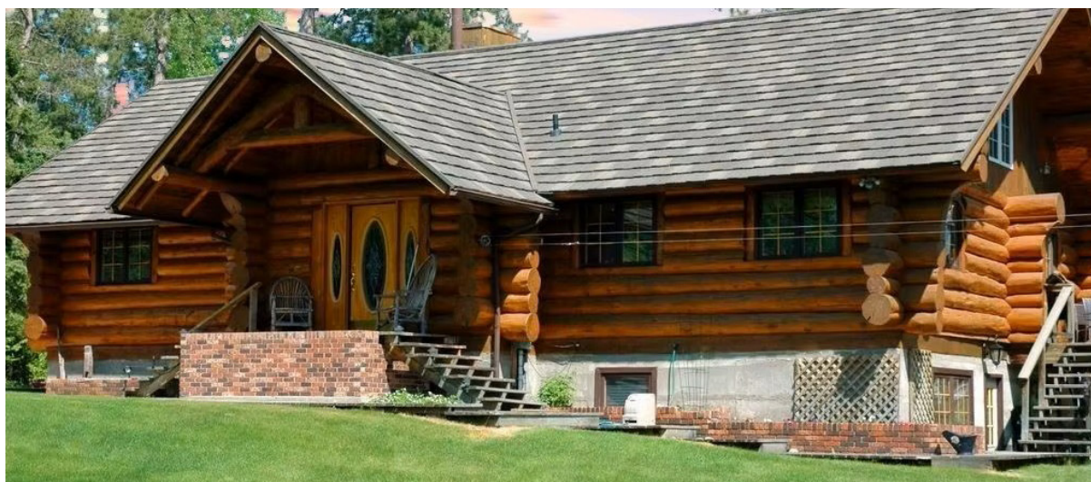
Figure 5.19.2: Picture of a Wood Shingle roof
