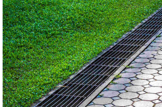
(B) Inlet surface drainage system
