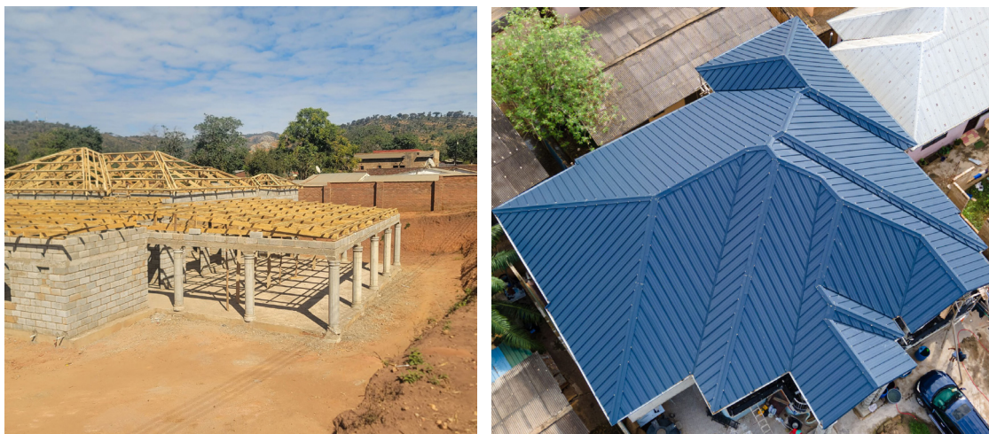
Figure 4.13.4: Roof carcass ready for roof and final finishes applied to roof carcass.
