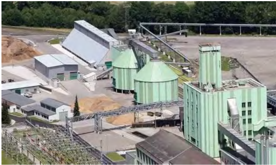
Figure 5.10: Picture of Bioenergy Storage System
