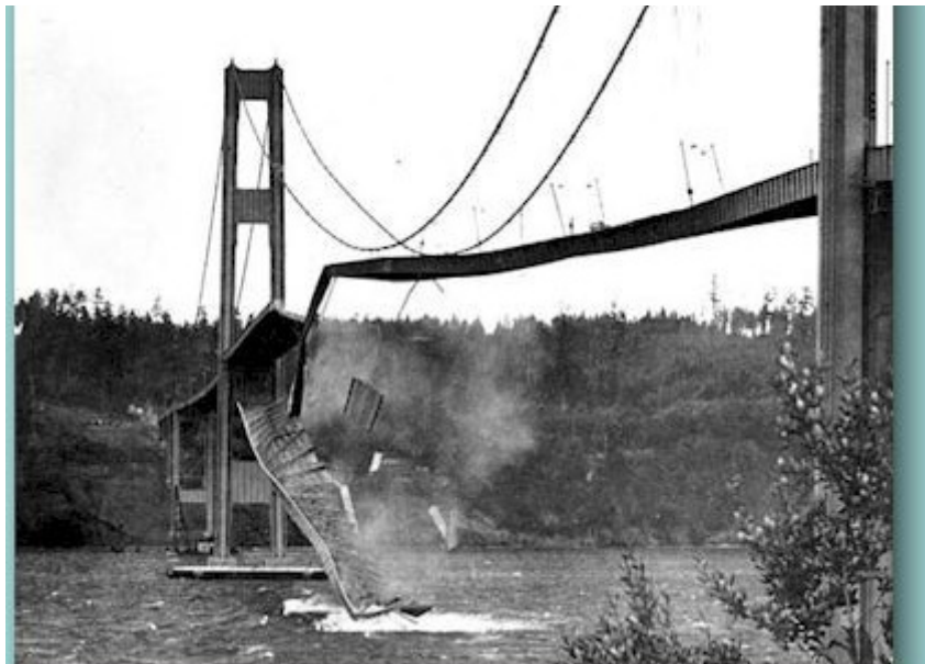
Figure 2.17: Tacoma Narrows Bridge twisting https://lib.uw.edu/specialcollections/collections/exhibits/tnb/collapse/
