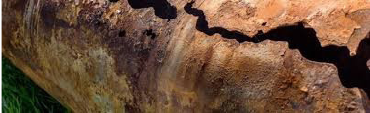
Figure 2.15: Failure resulted from the rusting of steel in humid conditions
