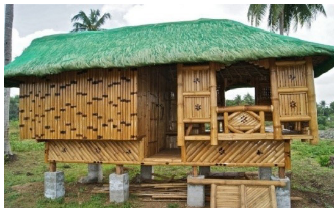
Figure 2.8: A housing structure made of bamboo
