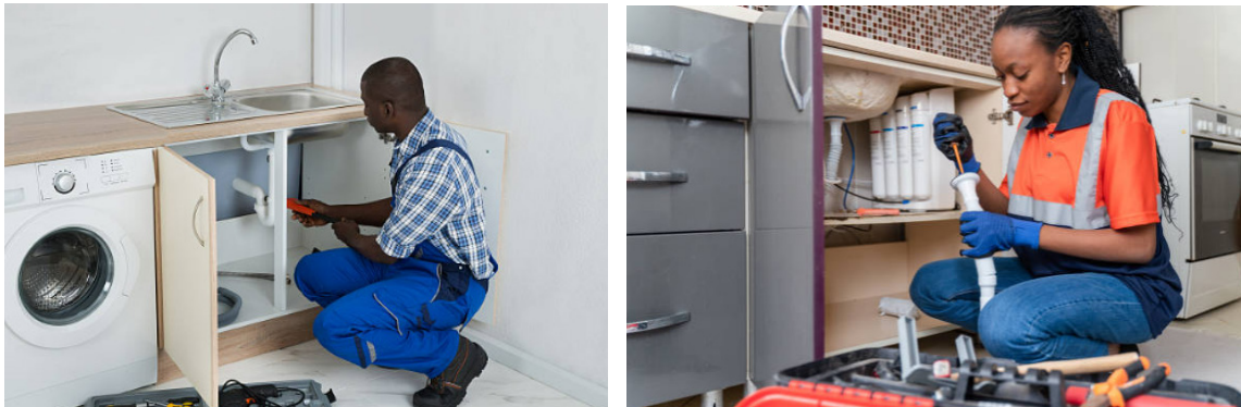
Figure 4.17: Care and Maintenance of Household Water Supply by Professional Plumbers.
