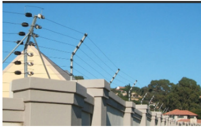
Fence with electric/wire protection
