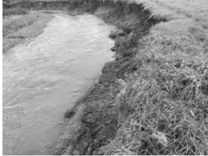
Figure 12.6: Stream bank erosion
