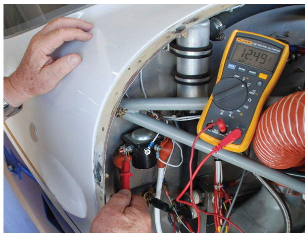
Figure 4.6: Multimeter testing power supply
